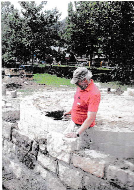
An overview of the substructure and wall surround. The clay in cente will be the coke oven floor
