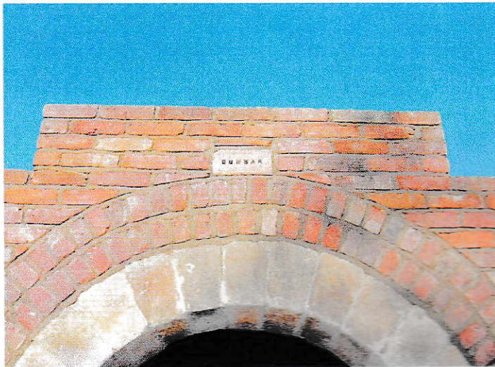
The Completed Arch & Position of the Dunbar Brick
